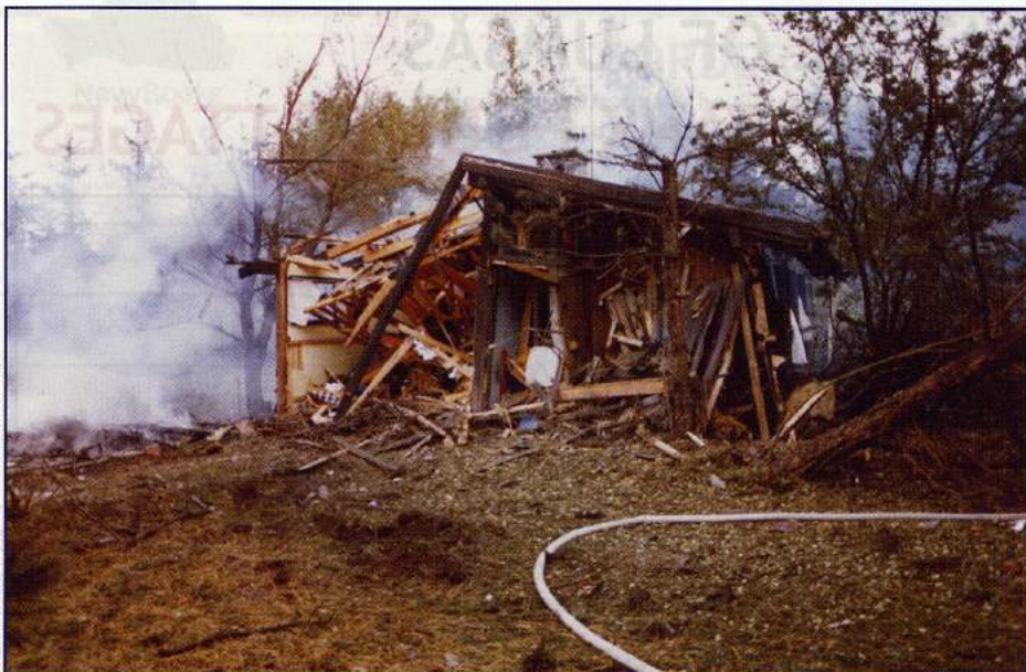
One of the destroyed summer cottages at Lumsås, 6. September 1982. Had the accident happened during a weekend in the summer, the houses would have been full of people on vacation. On a Monday in September 1982, most of the summer cottages were, luckily, empty.
